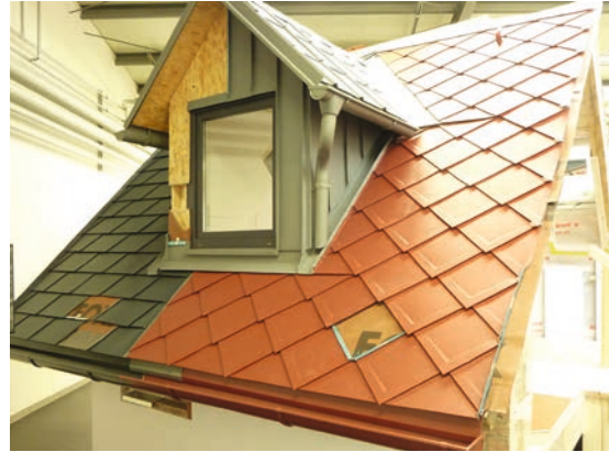
direct comparison between incorrect and correct execution of construction work
